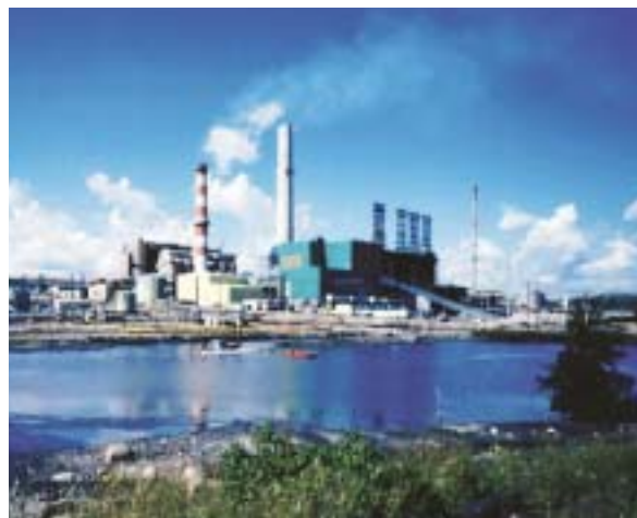
Suncor, Fort McMurray, Alberta, Canada. Extraction back pressure condensing application, 76.5 MW
